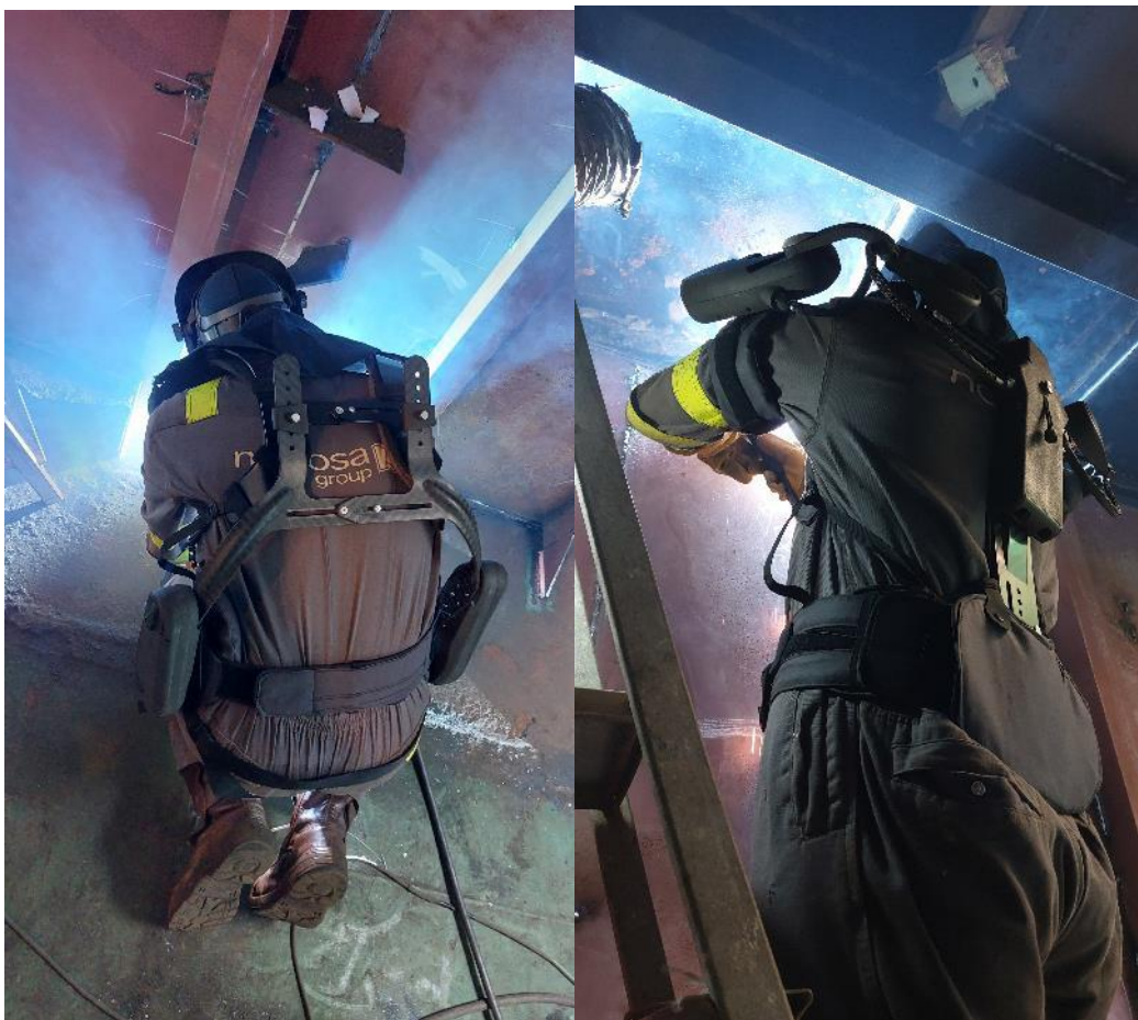
Figure 44. Workers using exoskeletons in welding activities (Vertical and Overhead welding positions)
