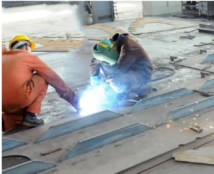
Figure 3 Current assembly and welding process performed by operators manually.
