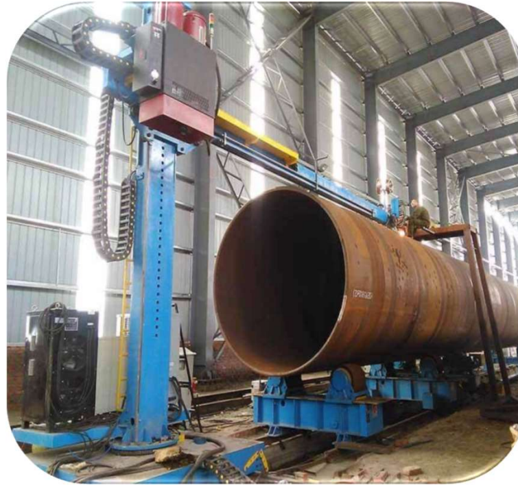
In Situ Wind Turbine Tower Repairs
