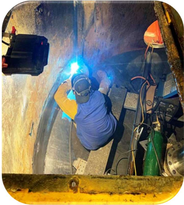
Manless Storage Tank Repairs
